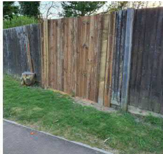
2: temporary gate installed by maintained land landscape contractor
