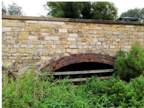
Culvert linking Tombs Meadow to the north end pond
